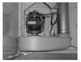
(9) Remove wires and 2 clamps that fix the motor bearing to detach the motor.
