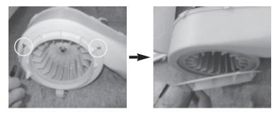
3. Separation of impeller fan: Fix motor axis and separate fan.
