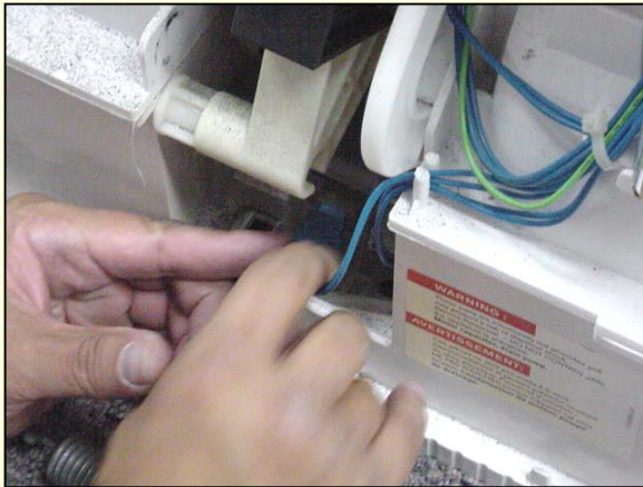
Disconnect drain pump wires
