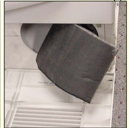
Remove front insulation
