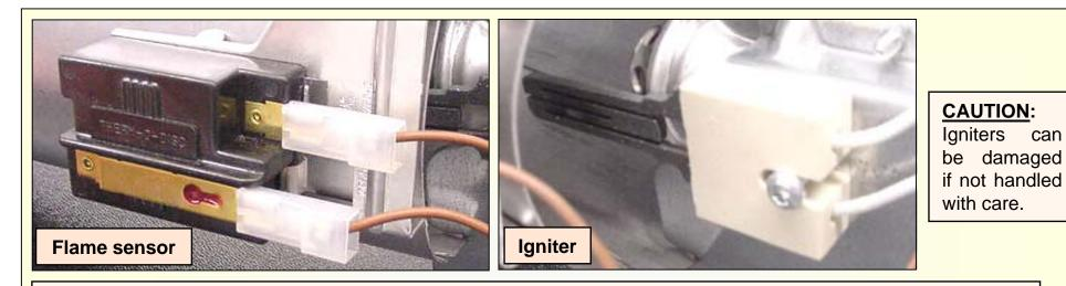
Flame sensors & igniters are each held in place by one screw. Flame sensors have a tab and slot – slide them up.
