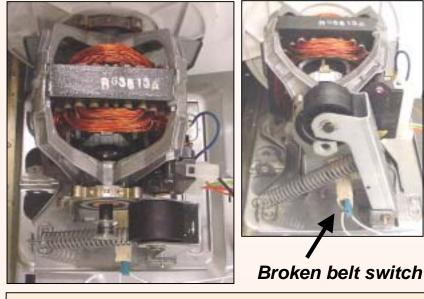
HINT: Remove rear panel to access drum drive motor, belt/pulley & electric heater/gas burner.
