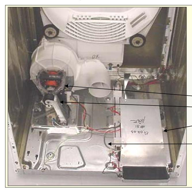
Electric dryer after drum has been removed.
