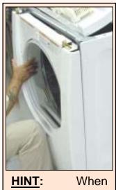
**<u>HINT</u>:** When aligning front panel tabs on frame, make sure door seal is seated properly.
