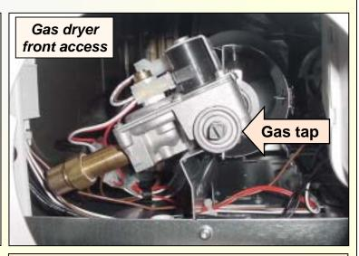
**HINT**: Gas valves and burners are attached together to a single bracket. To remove them, screws must be removed from the base and burner chamber.
