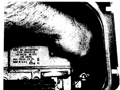
Internal gas shut-off valve
