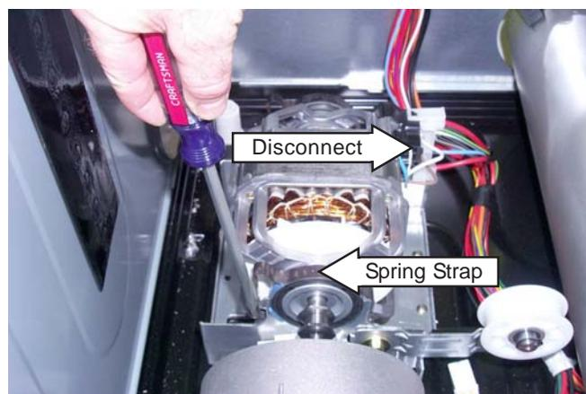
5. Remove the spring straps. Remove the drive motor from its cradle.
