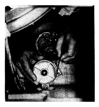
8. With the belt completely installed, feel with both hands to see that it is properly positioned in the motor pulley and in the approximate middle of the idler pulley. When you have determined by feeling that it is installed correctly, lift up and push back while slowly turning the tumbler one or two revolutions in a clockwise direction to allow the belt to properly align itself.
