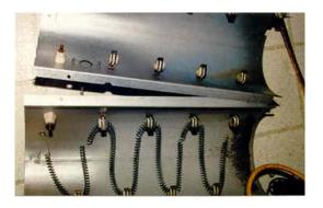
Electric elements are not interchangeable between brands. In contrast to the gas coil systems and igniters, each heating element is brand specific.
