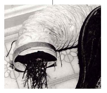
If the complaint is long drying time, advise a customer during the initial call. Ask them to check the vent system. A skilled mechanic doesn't really want to be too involved in taking down venting. Small jobs, yes, but often the task is more involved. Frequently, vents are built into a wall or finished ceilings and are virtually inaccessible.
