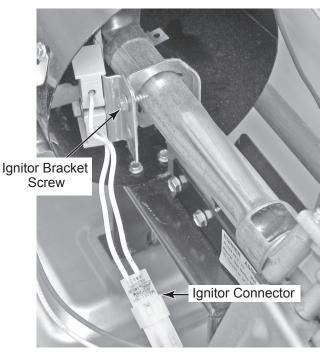
c) Remove the 5/16<sup>"</sup> hex-head ignitor screw and remove the ignitor from the bracket.
