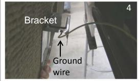
Lift the door up, and support the top of the outer door and ease the bottom of the door out towards you. Reach underneath, disconnect the ground wire from the bracket and lift up on the bracket slightly to clear the rim of the tank.
