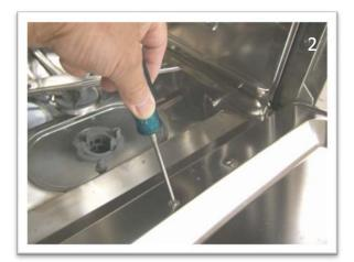
Remove the 2 bottom screws first
