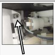
**<u>HINT</u>:** UC/12 model condensation tubes exit in the base behind the sump. There is <u>no</u> drain connection for these tubes. **HINT**: Vented dispensers cannot be used to replace unvented dispensers. If they are, dishes won't dry properly and there can be water leaking inside dishwasher doors.
