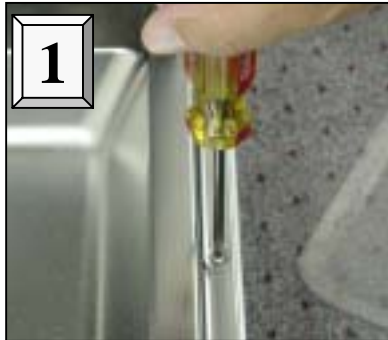
1 Removing door & fascia
