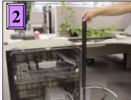
Removing trim strips
