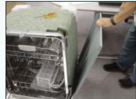
Lift panels up and out
