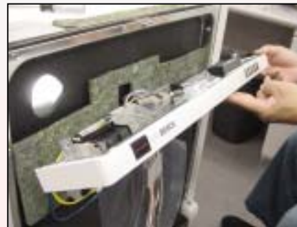
Replace fascia panel
