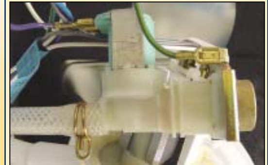
Removing hose clamp
