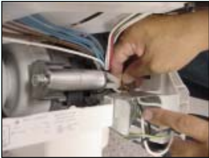
Pull wires from J-box
