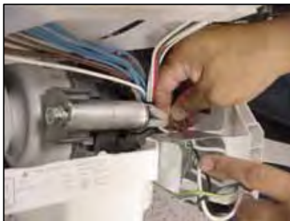
Pulling J-box wires
