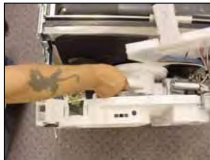
Pulling out sump hose
