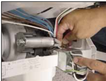
Pulling J-box wires
