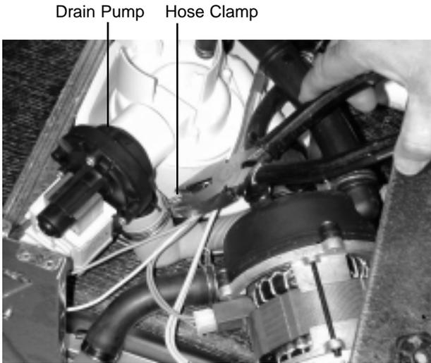
**5.2.34.4** Remove single Phillips head screw which retains Drain Pump to the sump socket as shown below.
