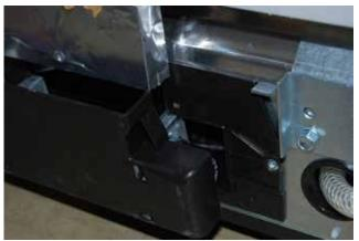
Pull blower assembly out towards you slowly as shown above. Disconnected blower motor connection as shown below.
