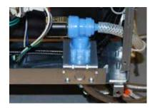
Remove the two screws shown above and remove the fill valve from the base.
