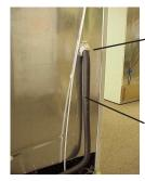
Push the heat exchanger through the hole in the cabinet.
