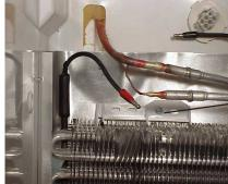
Remove the heat shield and reinstall the evaporator clamp.
