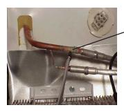
To replace the evaporator, cut suction line at this point.
