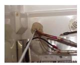
Using the permagum provided in kit, seal hole and end of old heat exchanger.
