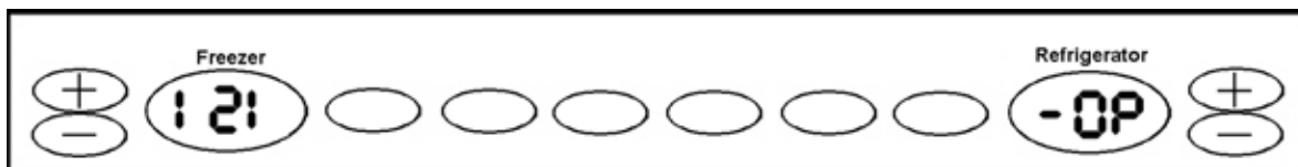
DAMPER IS IN THE PROCESS OF OPENING
