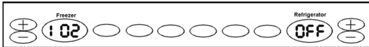
OBSERVE COMPRESSOR &amp; CONDENSER FAN FUNCTION
