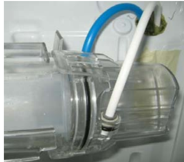
Hoses are accessible once tank is removed.
