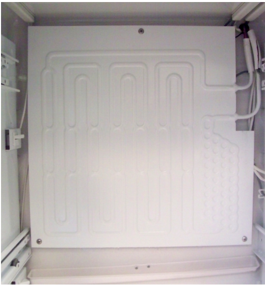
Figure 4.9: Evaporator plate used in the RF24D
