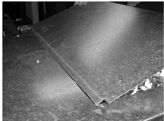
Replacing the Access Panel
