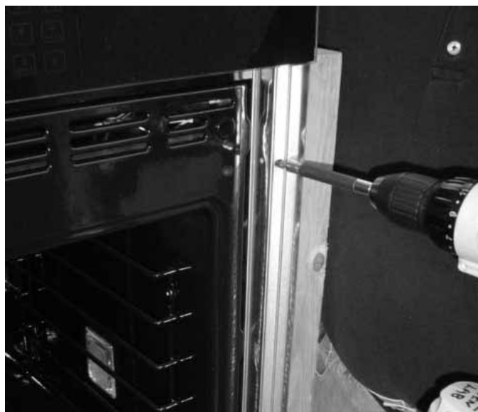
Oven Mounting Screw Locations
