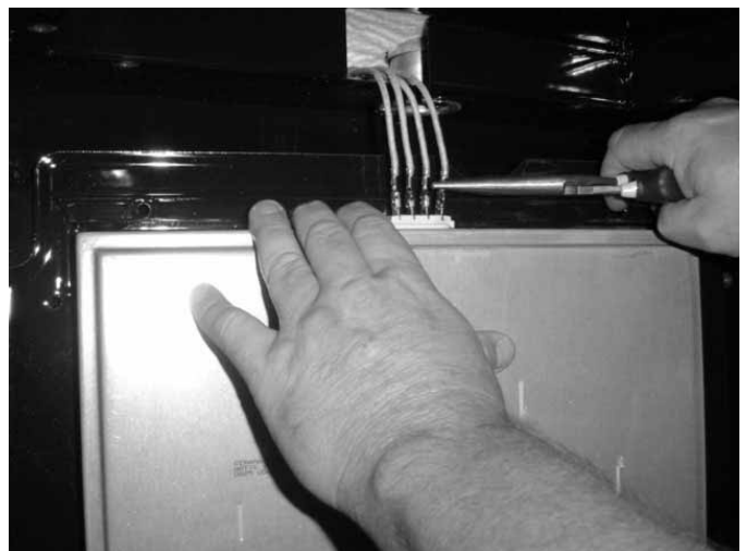
Connecting the Broil Element Wires
