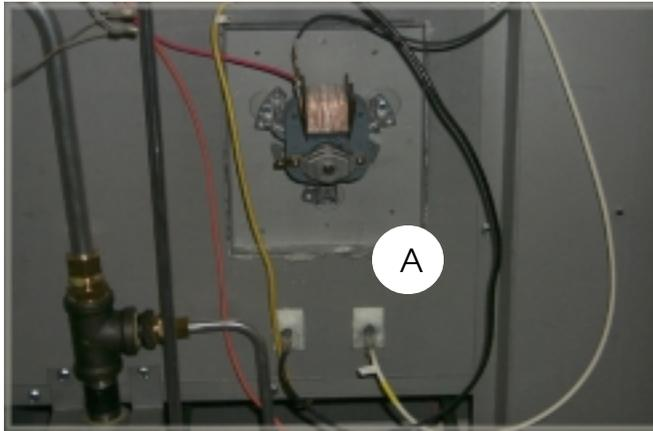
Figure 22-1 shows the convection motor part number (A) mounted on the outside, back of the oven
