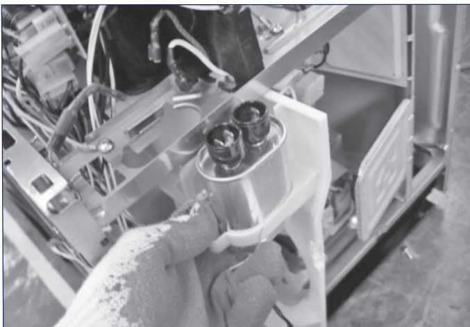
Figure 4-8. High Voltage Capacitor Removal
