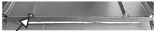
One screw at the bottom
