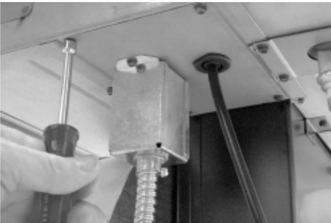
5. Remove the 1/4-in. screw from the bottom of the manifold and remove the valve.
