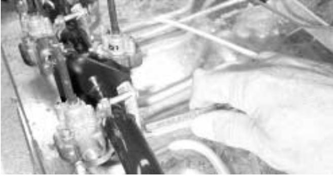
6. From under the counter, remove 2 screws at the manifold.
