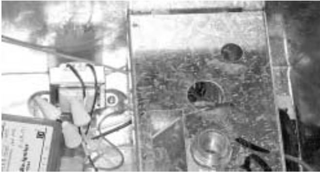
4. Remove 2 screws and the transformer.
