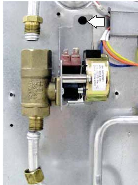
5. Disconnect the wires from the lockout valve.
