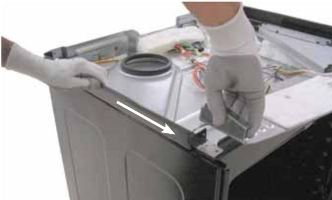
12. Remove the two 1/4-in hex-head screws from the back of the side panel.
