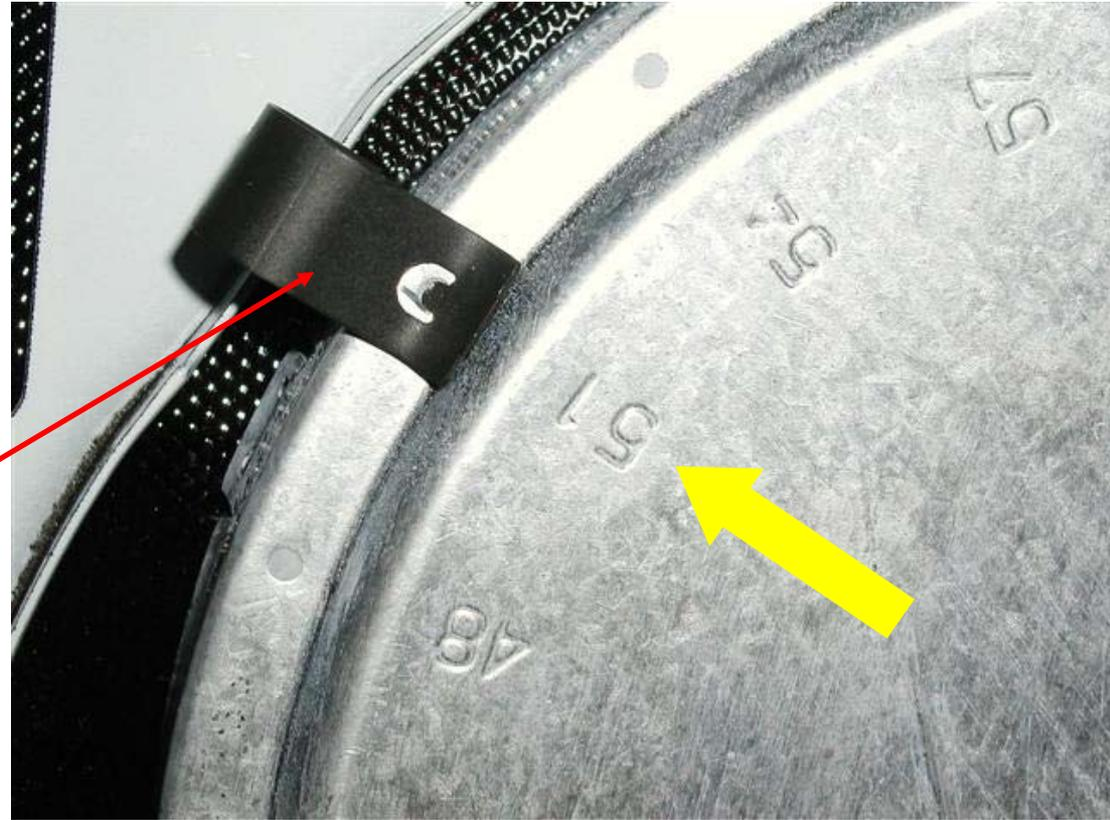
After marking the numbered holes on the burner outer case, lift up on spring clip to disengage it from the burner.
