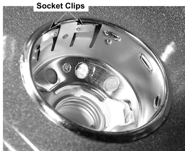
5. Disconnect the wires from the socket terminals.
