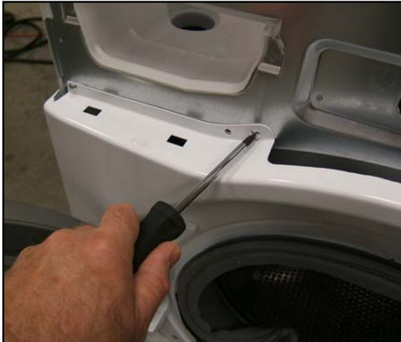
10. Remove 4 screws at top of panel
