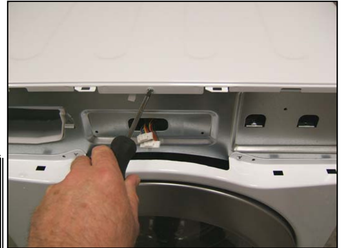
2. Remove 3 screws from front of cover
