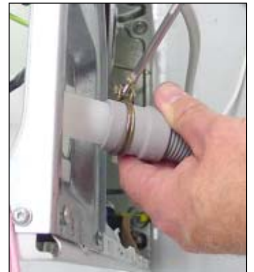
Disconnect drain hose
