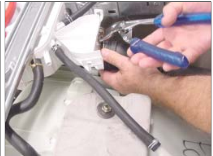
Remove door seal Disconnect main water inlet hose Disconnecting main water inlet hose
