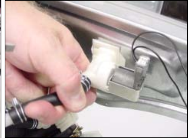
Disconnect hot water valve hose
