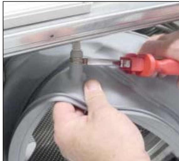
Remove door seal Disconnect main water inlet hose Disconnecting main water inlet hose
