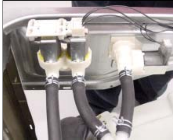
Disconnect water inlet valve hoses
