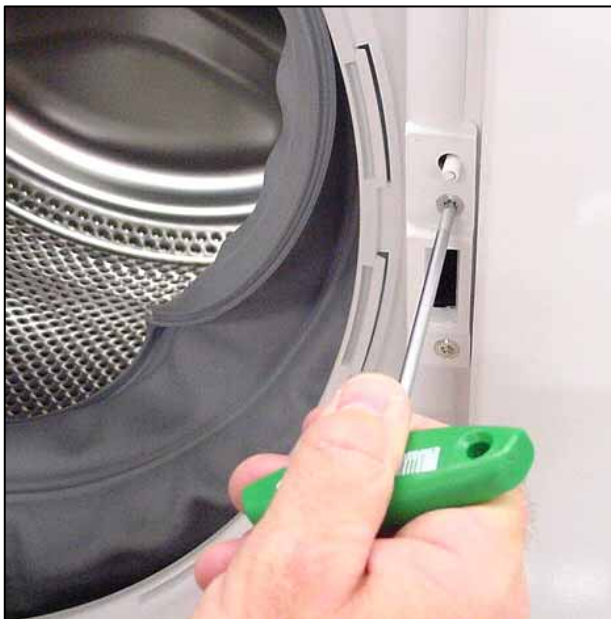
Remove door latch screws
