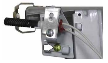
The flame detector is attached to the left side of the combustion chamber.
