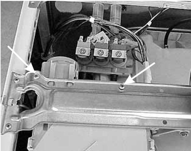
6. Remove the (2) screws holding the housing to the console panel.
