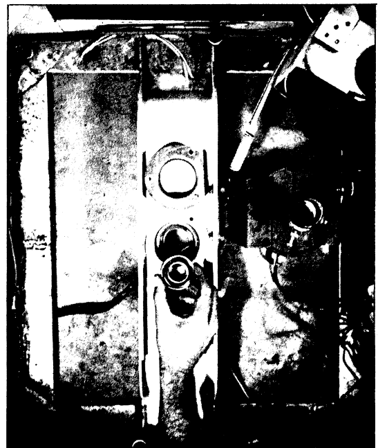
Figure 95 - Replacing Radial Bearing
