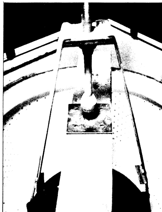
Figure 132 - Removing Stuck Agitator
