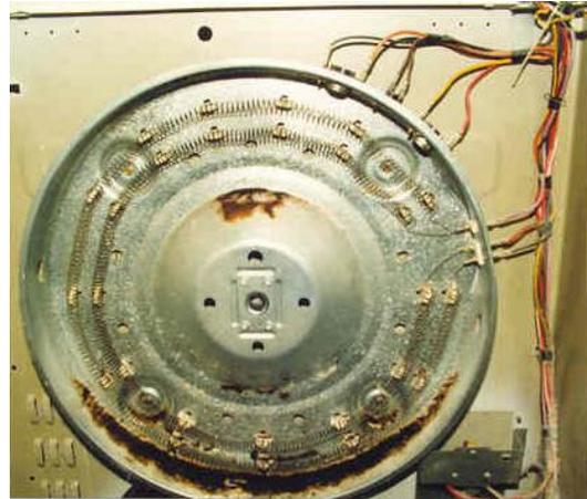
Burned out electric elements are commonplace. Burned wires at the high limit thermostat are also common. Virtually all dryers have a single coil heating element with two wires connected to it. GE is the only current exception. For many years, G. E. has had two independent concentric coils that supply the heat. One coil is used for low heat and both are used for regular or high heat. A few, very old Whirlpool dryers, also had a double coil system.
