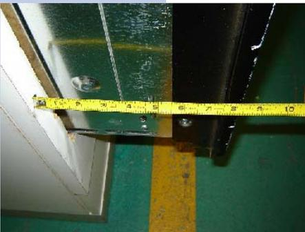
2.4 In order to replace the relay board and access the door lock assembly, you may need to pull the unit out roughly 8 inches in order to remove the front cover.
