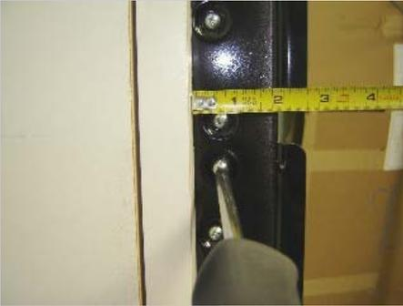
**3.11** Unlock the unit from its mounting brackets and pull the unit out of its cutouts roughly two inches.
