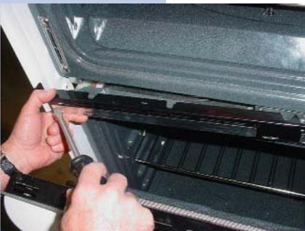
**3.14** You may use a flat screwdriver in order to release the center trim from between the two oven liners.
