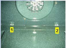
**12.5** In order to install the hidden bake cover, just align the 2 cover tabs through the 2 openings on the back of the cover.
