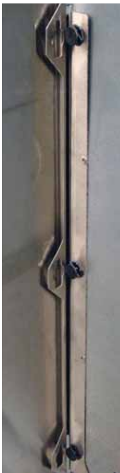
View Inside Panel
