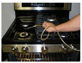
Measuring gas pressure can be easily accomplished at any of the 5 surface burners.
