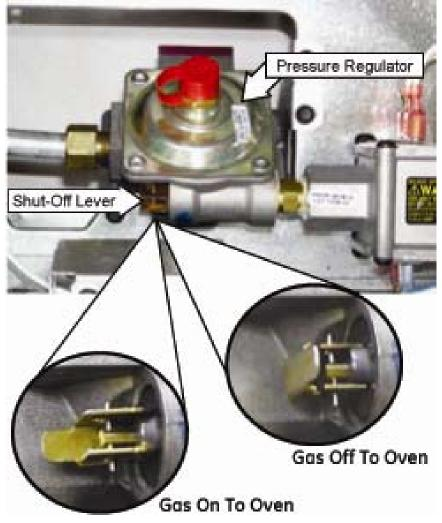
The shutoff valve allows servicing the oven burners without having to pull the range out and shut off the gas main.
