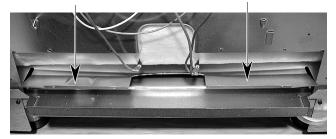
c) Use a pen knife or a single-edged razor blade and cut the insulation blanket, as shown. Be sure to separate the insulation blanket as cleanly as possible.
