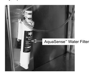
All tubing connections to the filter and hard connections are John Guest fittings.
