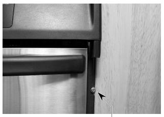
Cabinet Mounting Screw (2 Screws On Each Side)
