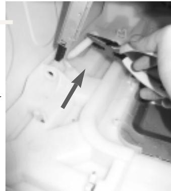
**3. Remove shock pin on tub side in the same way and remove the shock.**
