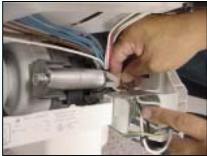
Pull wires from J-box
