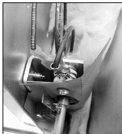
**Un-insulated terminal** (From Pilot Light) Placed on piggyback terminal
