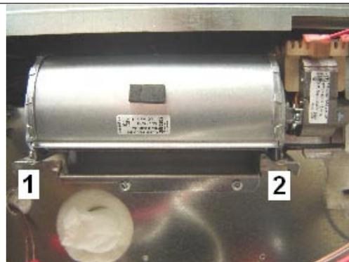
**11.13** Pull the cooling fan away from the unit and remove the 3 wires.
